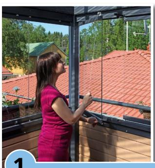
Push aside the pull knob in the bottom edge of the first panel. Pull at the string hanging from the upper latch and open the pane allowing it face the sidewall of the balcony. You may also leave the pane in the airing posi-tion if you want.
